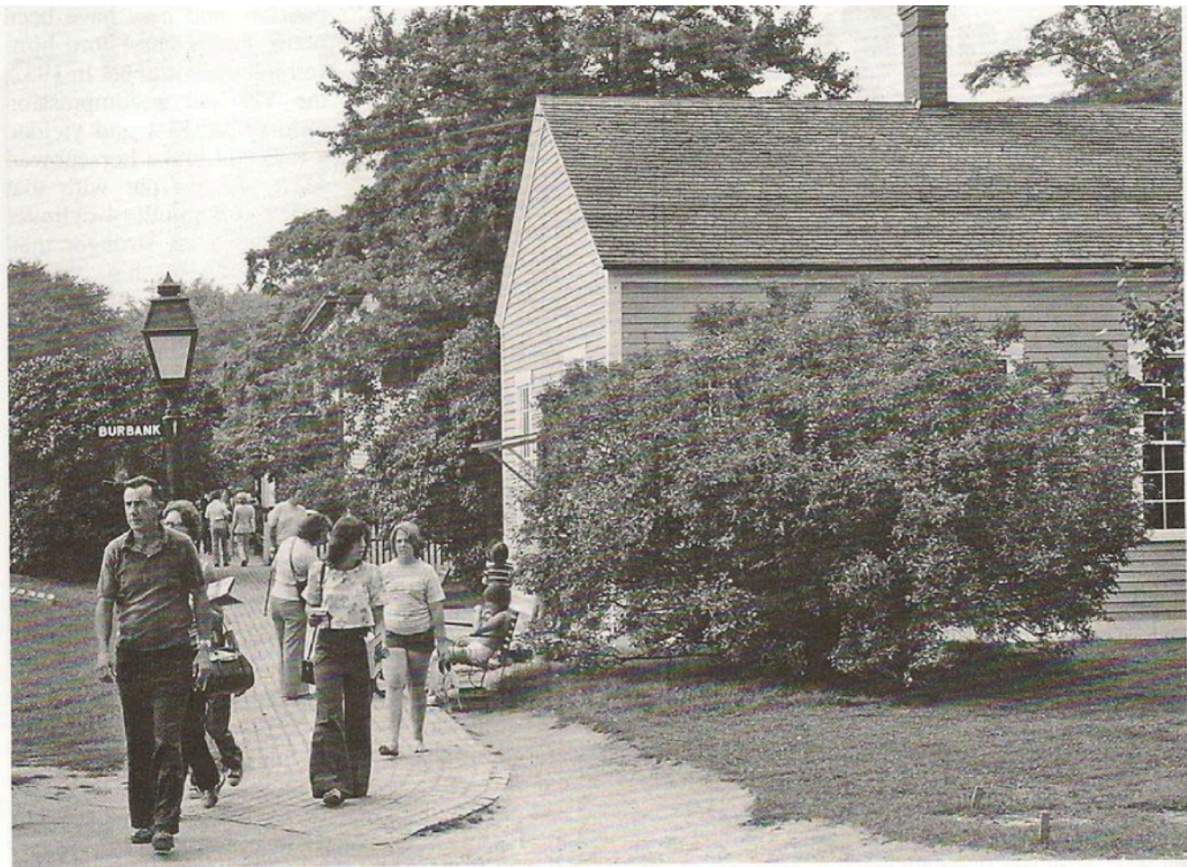
■ Visitors to Ford's Greenfield Village pay little attention to the Fort Myers laboratory, not realizing that this nondescript building was the site where the famous flathead Ford V-8 engine was designed. Photo by Charles Seims, 1973.
